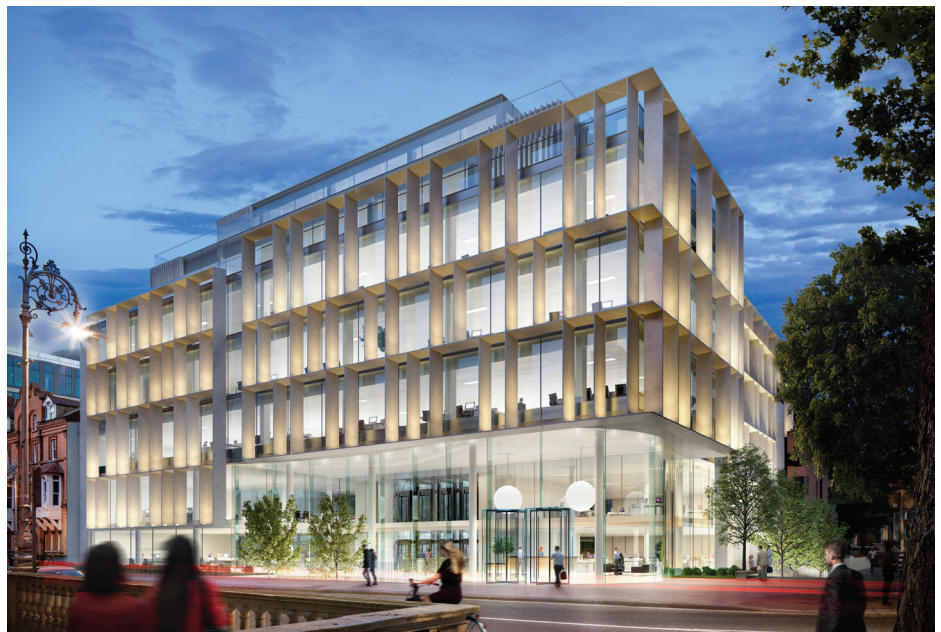
Earlsfort Terrace in Dublin exceeds NZEB requirements with natural gas
