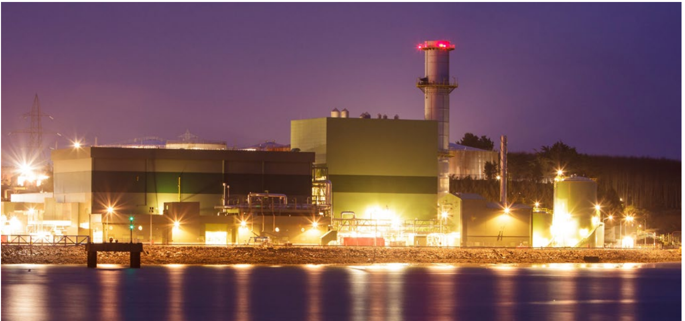
Figure 6-1 Great Island CCGT Power Plant
