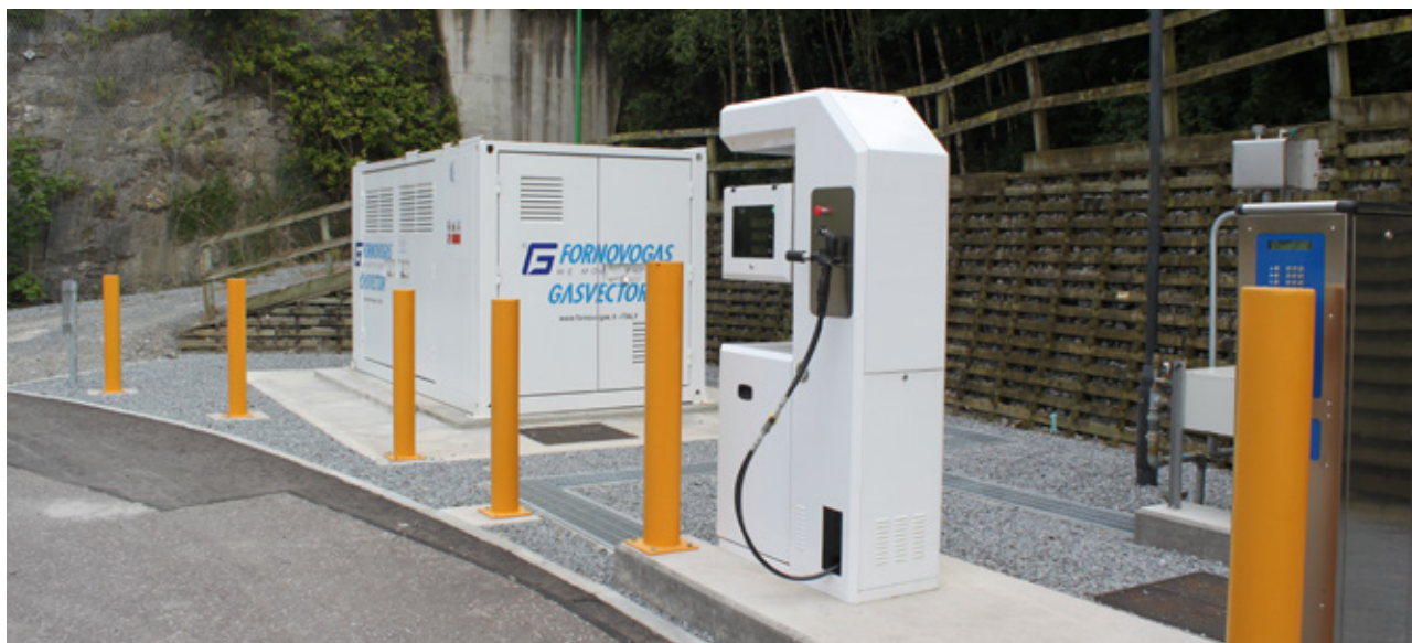
Figure 10.3: Bord Gáis Networks Fast Fill Station, Gasworks Road Cork
