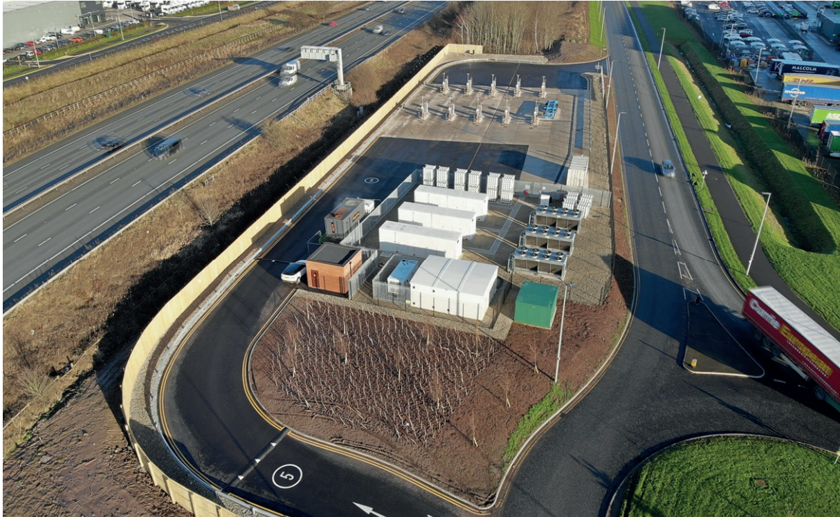
Figure 10: Example large scale CNG refuelling station operated by CNG Fuels in Warrington. Image courtesy of CNG Fuels
