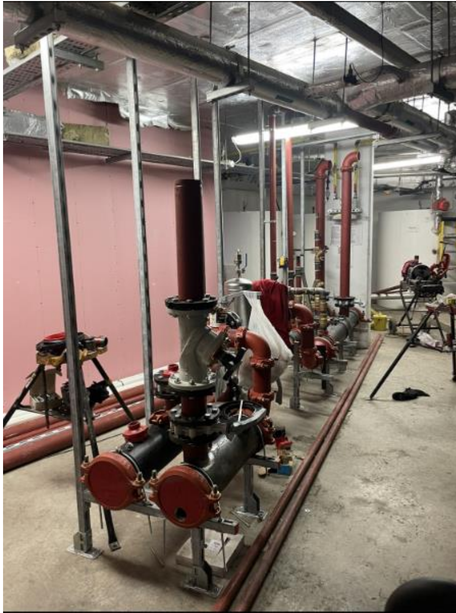
New modified header arrangement – mid installation
