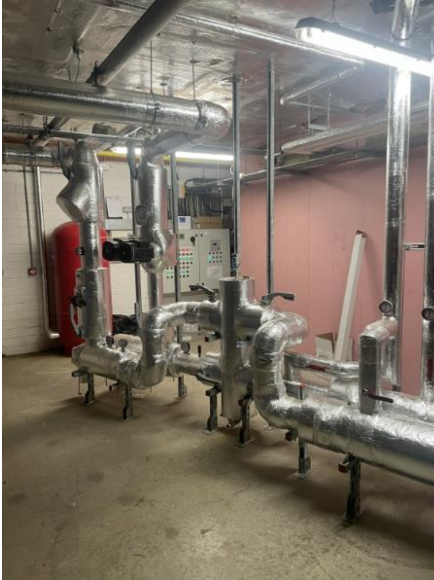
New header fully installed + insulated
