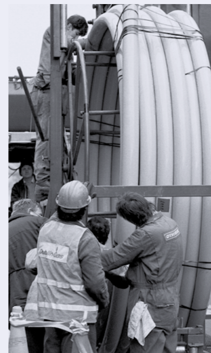
Dublin Gas Construction 1990
