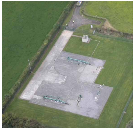
Figure 10.2 Aerial View of an AGI Site
