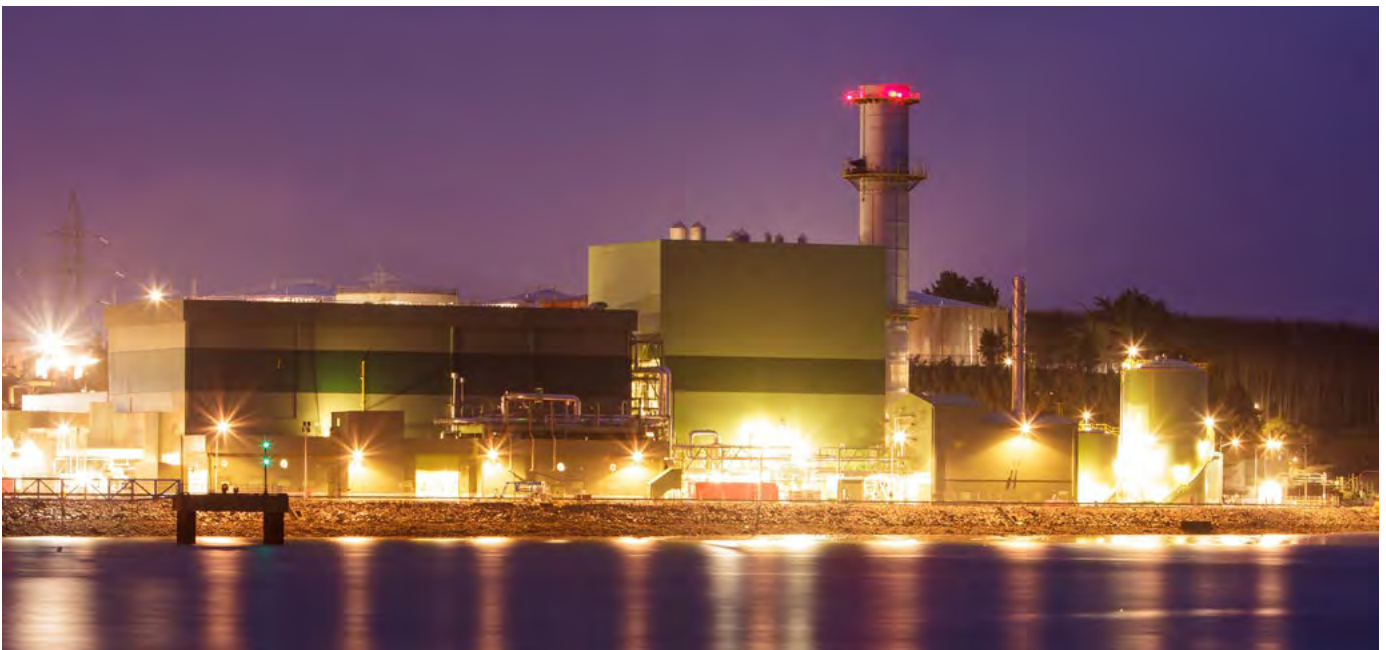
Figure 6-1 Great Island CCGT Power Plant
