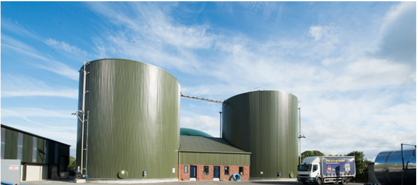
Figure 6-5: Green Generation, Nurney, Co. Kildare. First bio-methane grid injection project in Ireland
