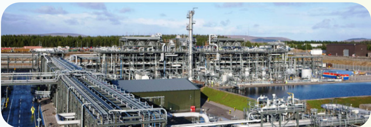
Fig 5.3: Bellanaboy Gas Terminal
