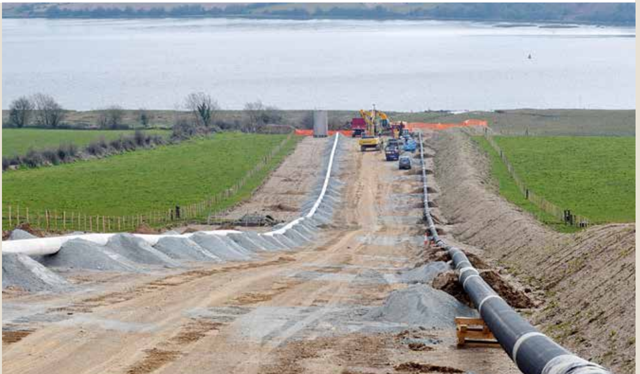
Pictured: Pipe string at River Barrow, Great Island, Co. Wexford
