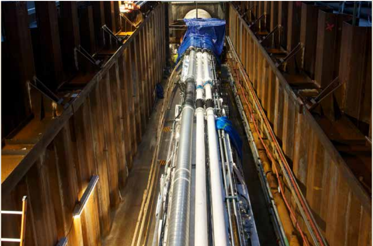
Picture: Tunnel boring machine in the shaft; Corrib Gas Project
