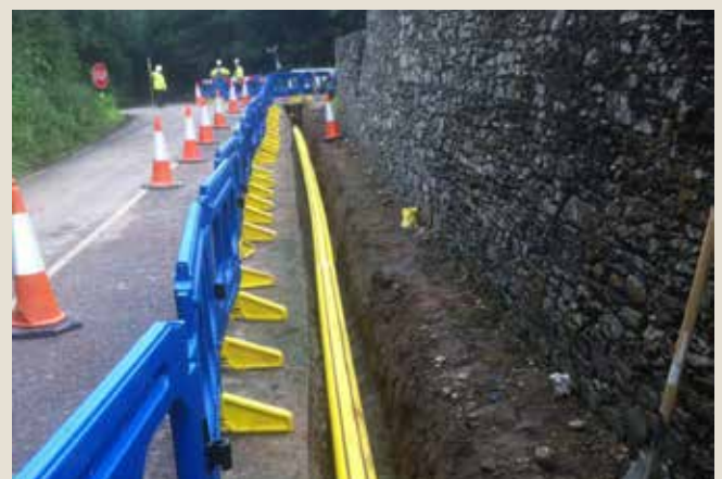
Pictured: Gas feeder main connecting Macroom to the natural gas network
