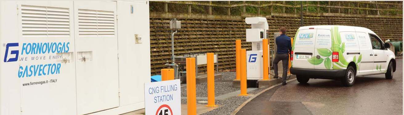
CNG Filling Station at Gasworks Road, Cork
