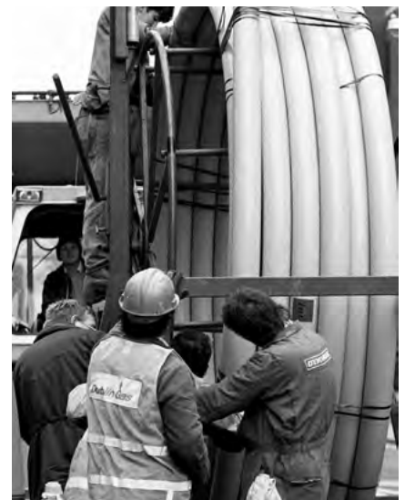
Dublin Gas Construction 1990
