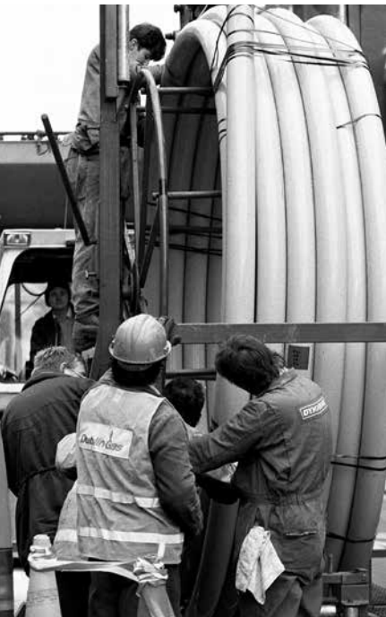
Dublin Gas Construction 1990
