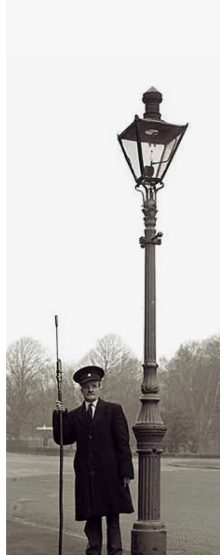
First gas street lamp
