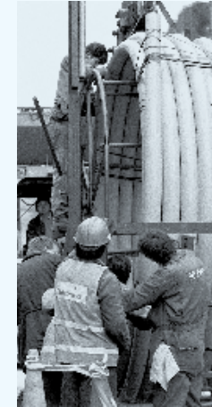
Dublin Gas Construction 1990s
