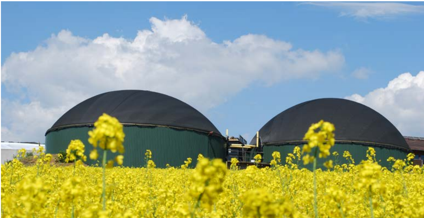
Anaerobic digestion facility
