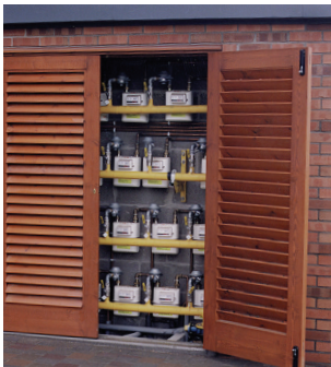
Purpose built multi-meter house (apartment complex).
