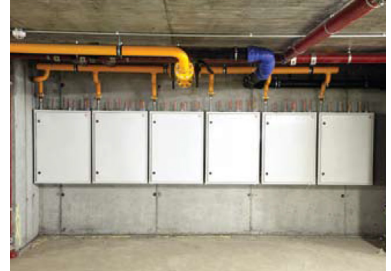
Top entry cabinet pre-fabricated off site
